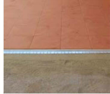
3. Lay the LINKedge at the edge of the pavers after removing excess paving sand. Assess how many EDGEspikes are required to lock pavers into firmly.
