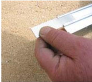
5. Connect any further 3m lengths together by using the provided fishplate.
