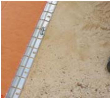
7. Once satisfied with the positioning of the LINKedge, hammer spikes firmly into the ground using a hammer. **Locking the pavers in place.**
